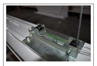
Fix the winch steel cable to the mounting system as shown in the picture left.
