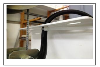
Cut the power cable of the electric screen to the desired length and fit it into the power connector box together with the output power cable of the cable coiler.
