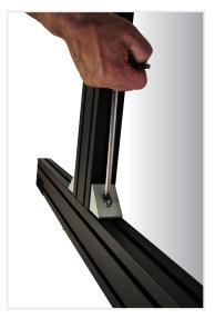
Mount the vertical part of the floorstand to the horizontal part that goes on the floor.
